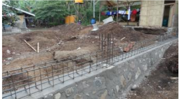
The chapel foundation
