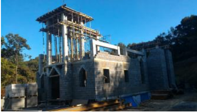
Walls waiting for a roof in Nakhodka
