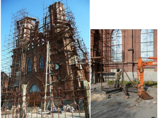
The brickwork for the two steeples is now done, except for some trim. The interior woodwork still remains to be done, and hanging the four bells. Now we are working on the final upper pointy parts of the steeples. You can see the gray "mast" standing between the fence and the church. That is the very inner part which will be clad with metal and a cross placed on top to complete the steeples, once it is lifted up and placed on the brickwork.
