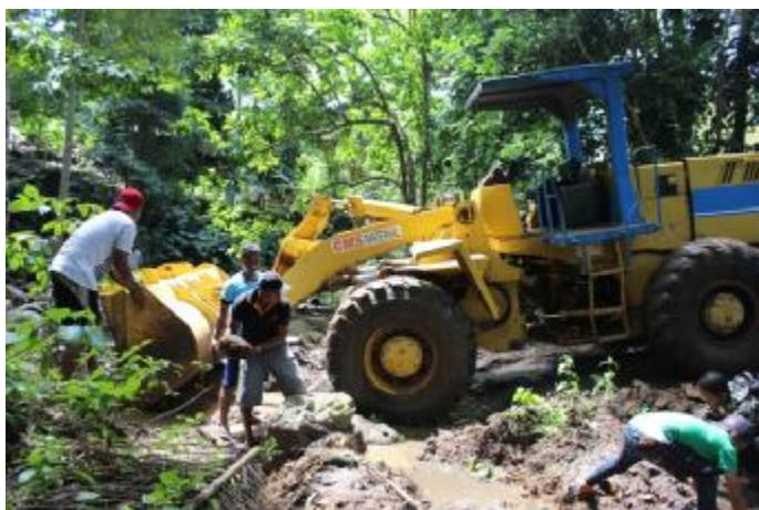
The bulldozer making a road to our land.
