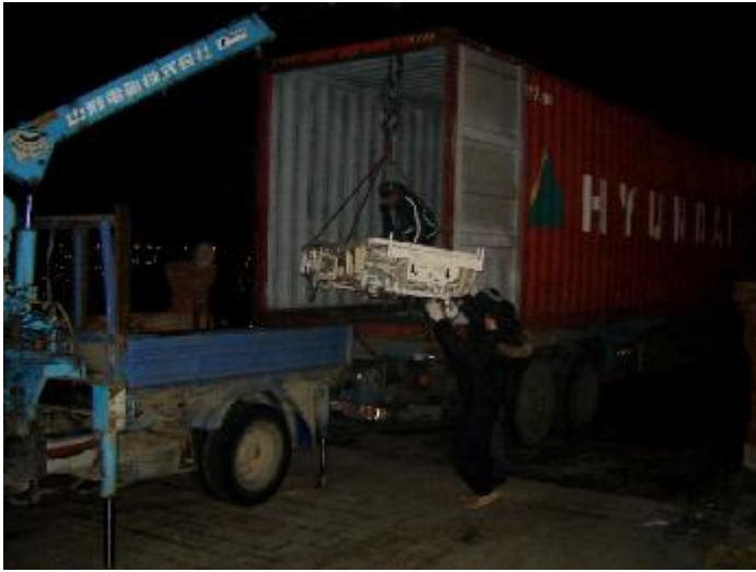
Even with a crane, it was a tough job.
