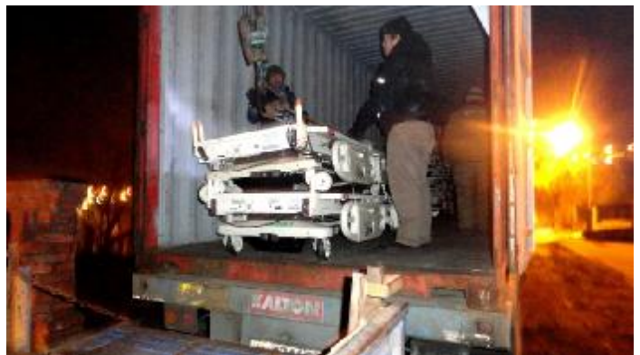
We had a crane to remove the heavy beds from the semi.
