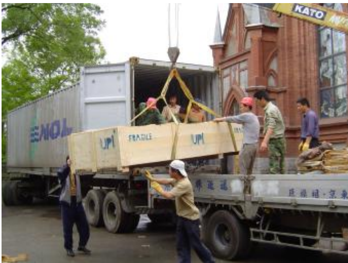
Unloading the roof and organ parts in the courtyard.
